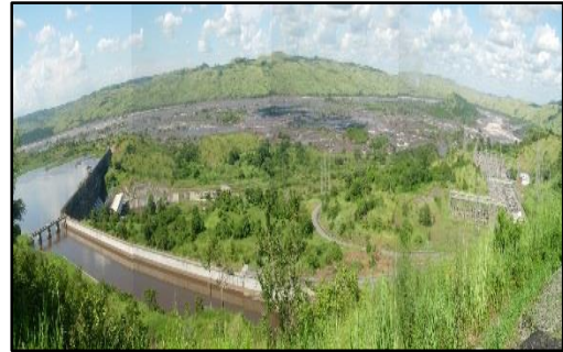
Inga Dam (Source: Internationalrivers.org)
